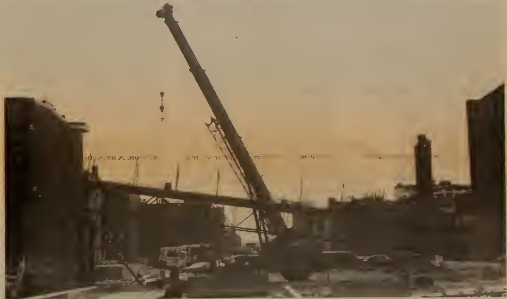
Dismantling of West Canton Street temporary pedestrian bridge.
